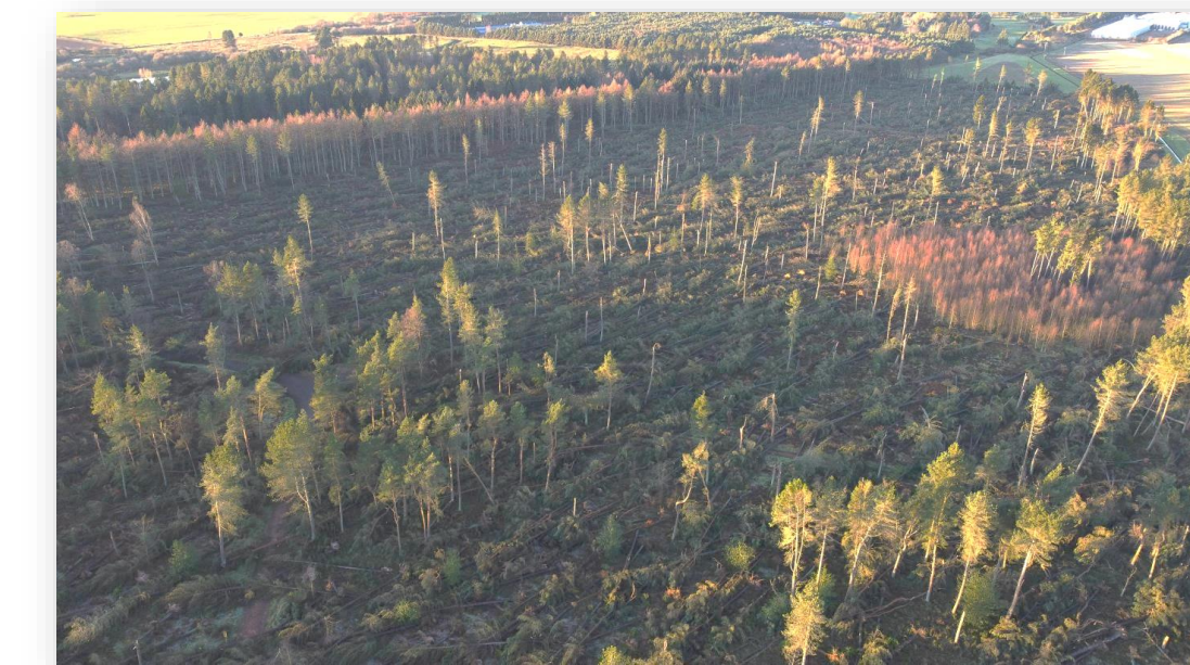
Figure 1. Tentsmuir Forest on April 2022. Thousands of trees uprooted, tons of wood lost, an enormous damage both for landscape and forest business
